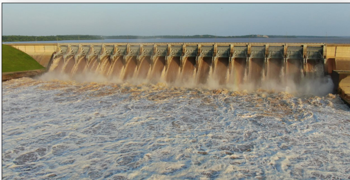
Large volumes of water released from a dam can cause flooding downstream. Some maps available on the National Inventory of Dams (NID) show this scenario. (Keystone Dam, Oklahoma)
